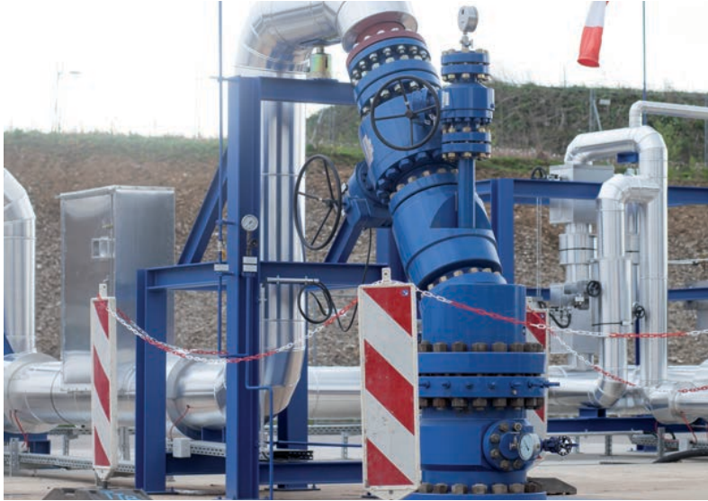
Blue colored wellhead by Hartmann for the injection well.
